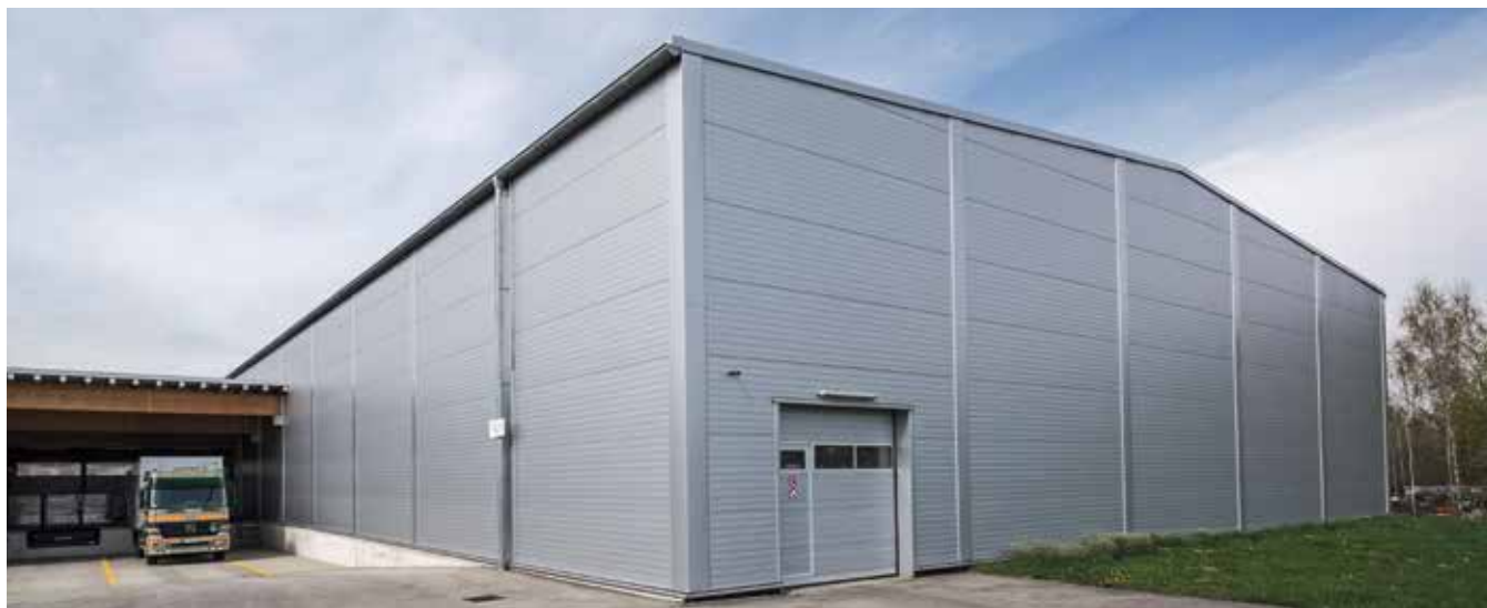
Horizontal laying – screw heads are covered by pilasters.
